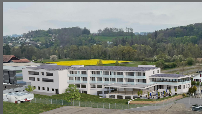
Airport Hotel Restaurant Bern-Belp
